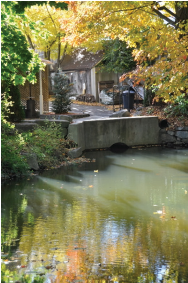
A culvert in Portsmouth's South End is close to overflowing during King Tide, October 2014. Photo by Cindy Jupp Jones.
