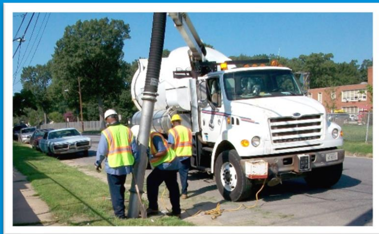
CATCH BASIN CLEANING
