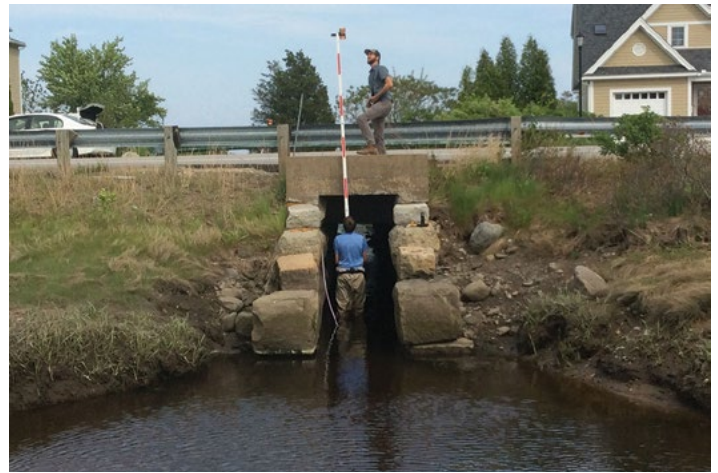
Figure 8: Surveyors plan a culvert restoration in Rye, NH, as part of the “Resilient Tidal Crossings” project. Designs call for this 3.5-ft wide culvert to be replaced in 2024 with a 15-ft wide structure, restoring natural hydrology to critical salt marsh habitat on the Seacoast. Photo by Kevin Lucey
